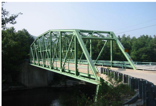
Gilead Bridge, NH
